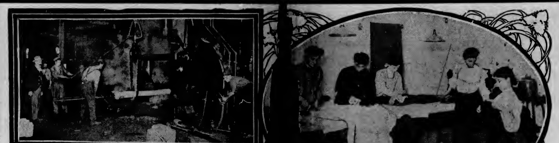
HAMMERING STEEL AXLE
